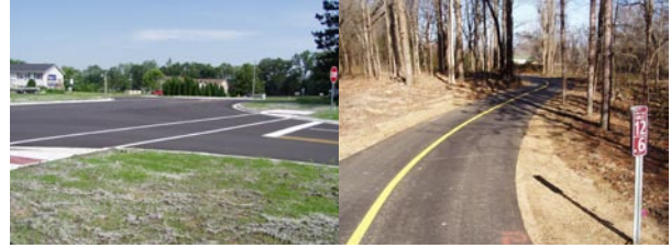
Pictured: Texas Drive Realignment and Kalamazoo River Valley Trail, Segment 2
